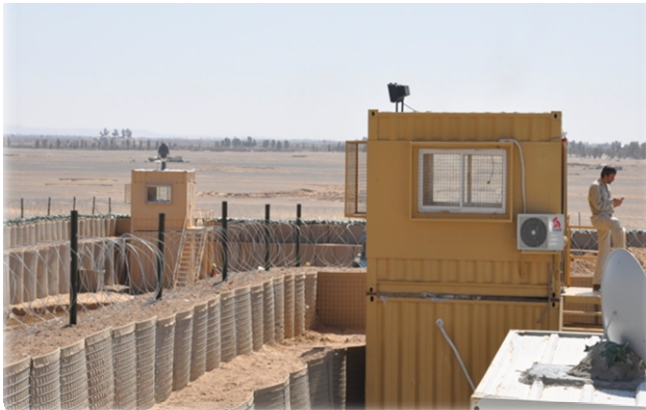
Picture 2 – Guard towers with HESCO Defensive Barriers
