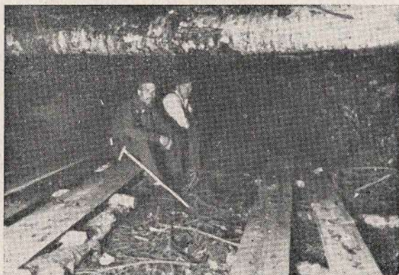
Sl. 42 — U bunkeru
